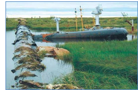
Uplifting of buried gas pipeline
