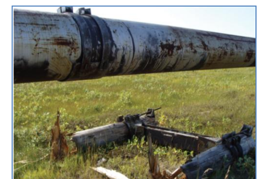
Subsidence of pipeline support (piles)
