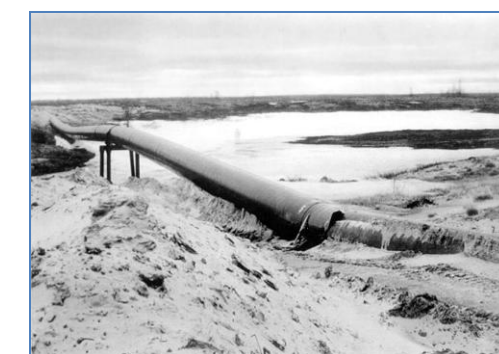
Frost heave of pipeline supports (piles)
