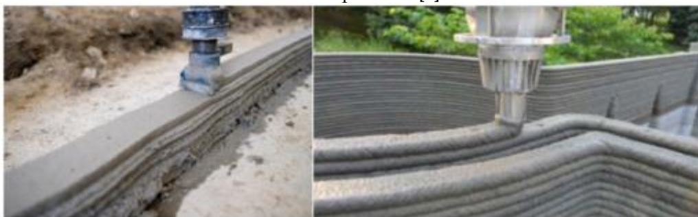
Pic. 1. Layering of building materials
