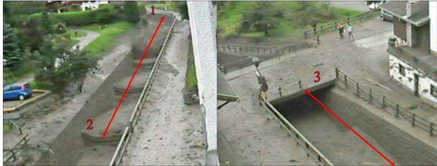
**Figure 4.** The scheme of the debris flow passage's sections: 1—step on the turn; 2—step in ridge of the parking; 3—bridge.
