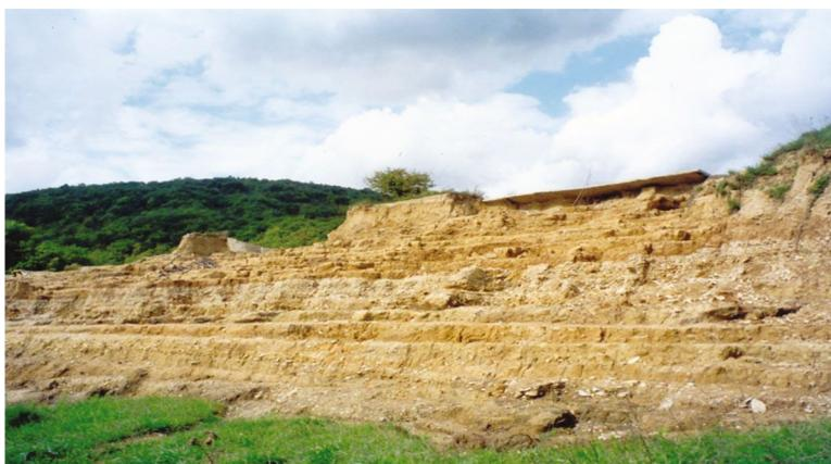
Fig. 1. The view of a half-destroyed dam from the downstream side.
