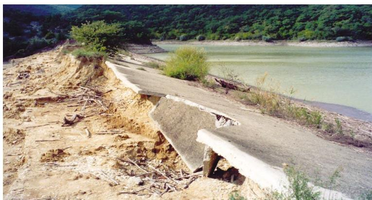
Fig. 2. The dam crest is washed out, but concrete slabs save it from complete destruction.
