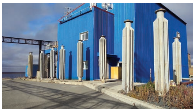
Figure 8.3. In Russia, thermosyphons are also often used to protect buildings, in combination with elevating structures on piles, such as with this building in the city of Dudinka (2018). Photo: Nadezhda Zamyatina
