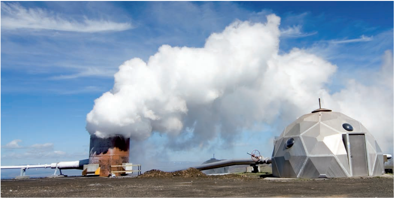
Nesjavellir geothermal power plant in Iceland. Photo: Crestock
