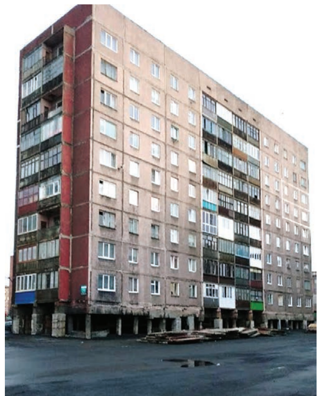
Figure 8.1b. The elevation of buildings (and other infrastructure) onto pillars allows for a ventilated layer between the structure and the ground, which helps protect against permafrost degradation: Norilsk, Russia. Photo: Nadezhda Zamyatina.
